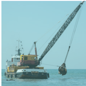
Dredging and Sediment Removal
